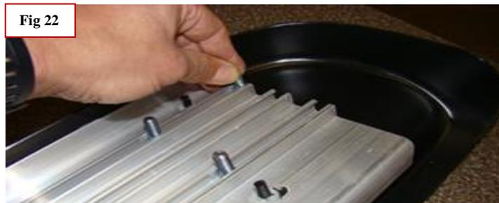
**Step 14:** Place the board on the installed mounting brackets. Align the bolts with the slots on the brackets and drop them into place. This is a tight fit and why the bolts from Step 5 (**Fig 12**) were left loose. Next thread the provided 5/16" flange nuts onto the bolts that hold the board and leave loose.
