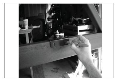
5. Use the supplied M10 Self-Tapping bolts to tap threads into the holes in the horizontal beam.
