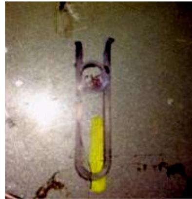
**Step 8:** Remove clip. Use a 1/2" drill bit and drill out the center mark. Slide the 3/8 clip back into position so the threaded part is aligned with the hole.
