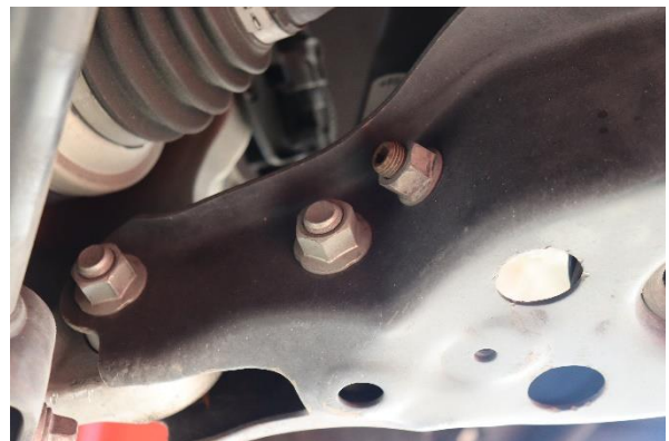
6. Remove the 19mm nut and bolt for the lower shock as well as the 17mm nut for the end link.
