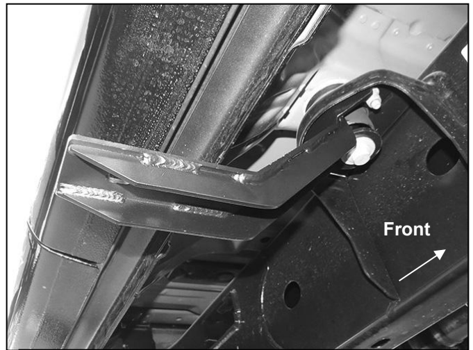
(Fig 8) Passenger/right center Bracket installed
