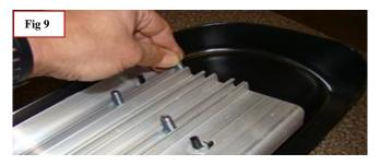
**Step 8:** Place the board on the installed mounting brackets. Align the bolts with the holes on the brackets and drop them into place. Next thread the provided 5/16° flange nuts loosely onto the bolts to secure brackets to the board (Fig 10)
