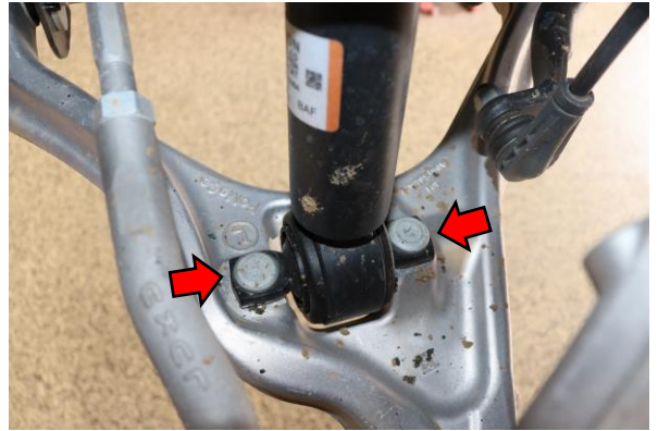
8. Use hammer to drive out both lower shock mount studs from the bottom. Applying heat to the studs can assist in their removal, be careful not to overheat the surrounding bushing or shock body.
