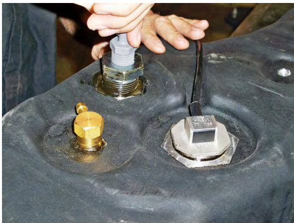
(Fig. 6) Installing 1/2" x 3/8" Hose Barb Elbow into
