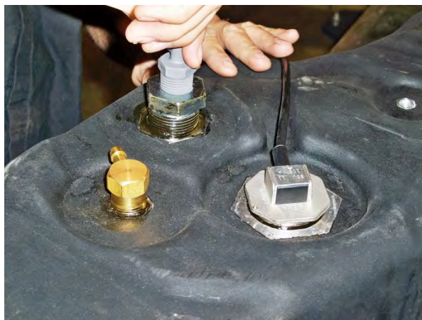
(Fig. 6) Installing 1/2" x 3/8" Hose Barb Elbow into plated Double Tapped Tank Bushing.
