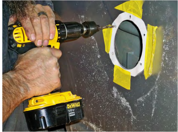
(Fig. 20) Cut out appropriate template and tape it around the 4.75" hole. Use center punch to mark screw positions and then using appropriate drill bit size, drill marked holes.
