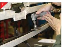
After both the upper and the lower sections have been removed. Sand all the cut areas smooth as shown above.
