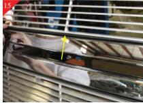
Place top billet grille into opening and center. Make sure to align with the face of the opening.
