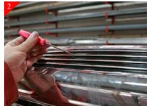
Place machined billet grille into opening and center. Make sure and check for alignment all the way around. Tape the machined grille in place using masking tape, so that it doesn't move during marking of the holes. Next mark hole locations using a scribe while using the machined piece as a guide to mark holes.
