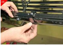
After drilling all hole locations place supplied U-clips on the brackets as shown.
