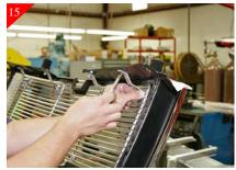
Using a scribe mark the mounting location where is meets the top of the shell as shown above.
