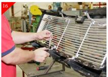
Using a scribe mark the mounting location where is meets the back of the shell as shown above. Make sure that the bottom brackets are firmly butted up against the black plastic shell before marking. Repeat for the remaining bottom bracket.
