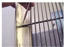
STEP 8 Locate & drill 5 1/8" holes in bottom of shell & atach using #6 x 3/4" self tapping screws. Re-attach arille shell. Installation is complete.
