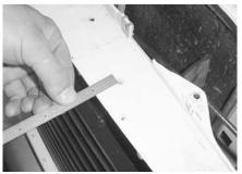
STEP 4 Mark hole location on top of core support 1" from the edge as shown.
