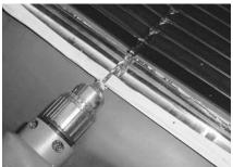
STEP 5 Set Billet grille into grille shell. Then mark center locations of each of the vertical rods of billet grille. Then drill a 1/8" hole at each location.
