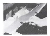
STEP 5 Set the grille in place in the opening and scribe around the vertical posts where they contact the frame.
