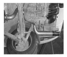
INSTALL THE OVERAXLE TAILPIPE #B INTO THE REAR OF THE MUFFLER AND USE CLAMP #E TO ATTACH TO MUFFLER. NOTE: TO GAIN CLEARANCE AT THE REAR OF THE BUMPER ROTATE MUFFLER CLOCKING AND TAILPIPE UNTIL YOU FIND THE POSITION WITH THE MOST CLEARANCE
