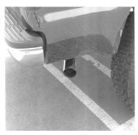
**6.** NOW INSTALL YOUR STAINLESS STEEL TIP. USE ANY ALUMINUM OR STAINLESS CLEANER TO POLISH YOUR TIP. THEN TIGHTEN ALL CLAMPS AND HANGERS.
