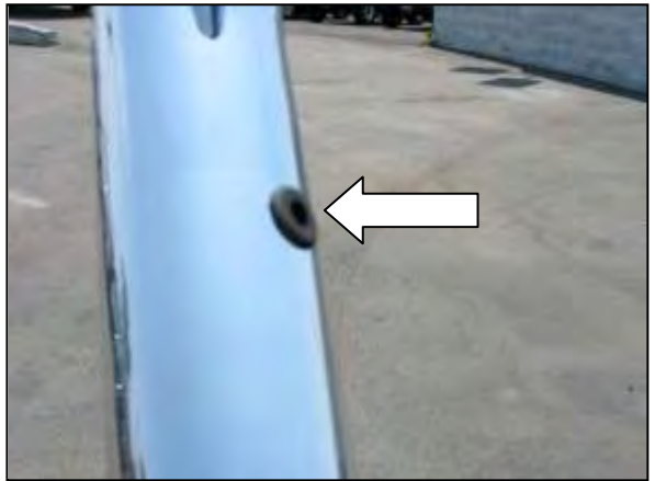
i. Insert the rubber grommet into the inlet pipe.
