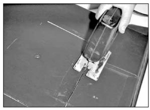
37. Using a jigsaw, cut along the horizontal and vertical lines.
