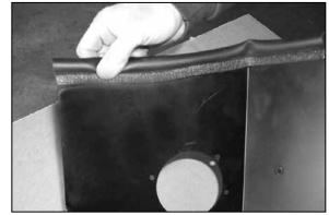
27. Install edge trim seal onto heat shield as shown.
