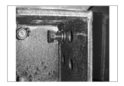
3. The backing plates do not have uniform hole placement and vertical orientation needs to be determined. Refer to for the proper orientation of the backing plate.
