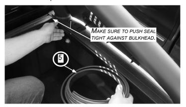
**STEP 4 CONTINUED:** What the side spacer seal should look like when applied up by the bulkhead.
